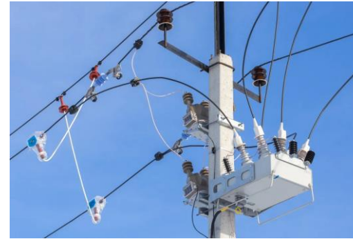
Digital Distribution Zones (304 reclosers, 263 motor-driven disconnectors)
