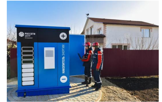
2 energy storage devices
